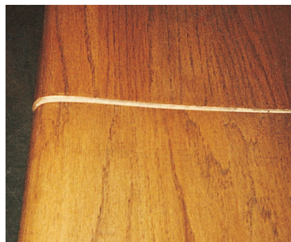
Avoid: misaligned seat joints (left) and pew backs (right) due to inferior butt joints.
