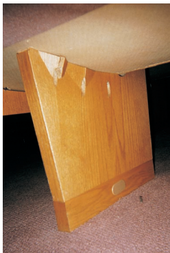
Avoid: inferior toe screwing method which causes wood to split from stress.
